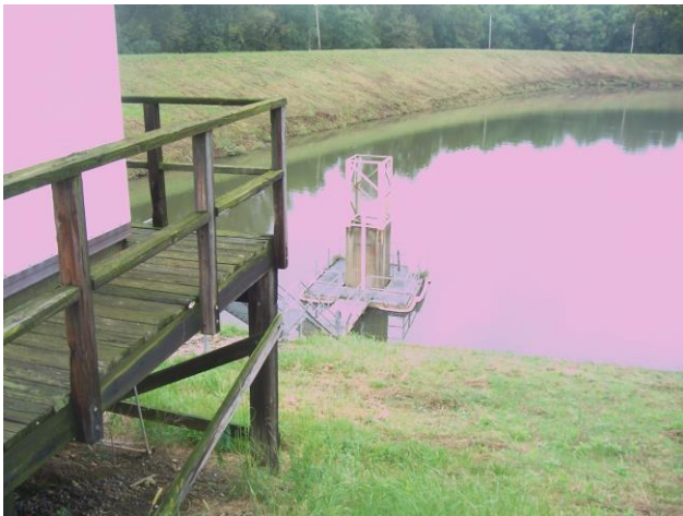
Photo 3 Typical view showing good conditions of the decant structure and interior embankment.
