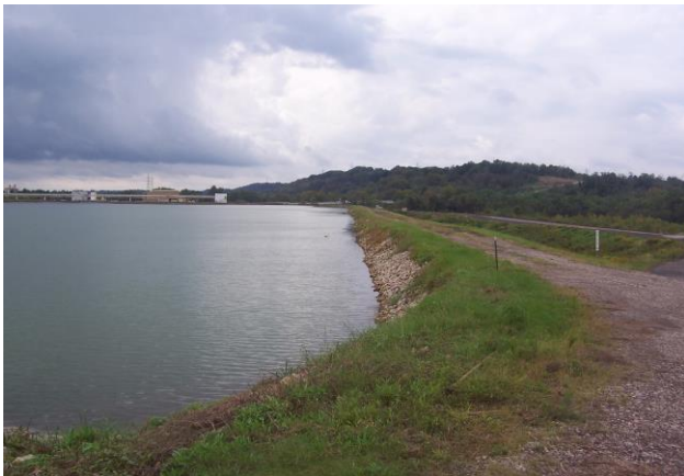
Photo 9 Typical view showing good conditions of the west embankment showing a uniform slope and crest. No erosion of the interior pond slopes was observed.
