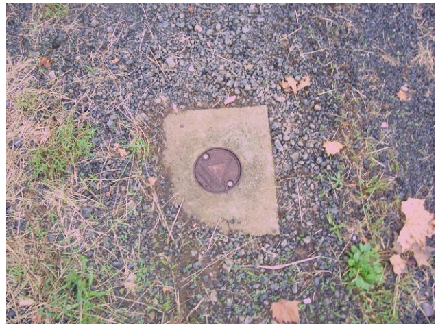
Photo 4 Typical view showing good conditions of the flush mounted piezometer installation showing the well cap seal and concrete pad.
