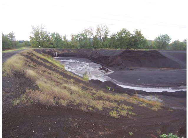
Photo 2 Typical view showing good conditions of the boiler slag embankment and stockpile of material to be used for beneficial utilization.
