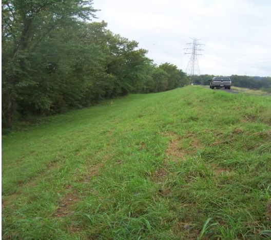
Photo 1 Typical view showing good conditions of the boiler slag embankment.
