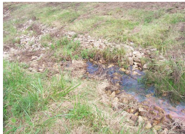
Photo 12 – Typical view of seep along the south dike showing a visually clear discharge.
