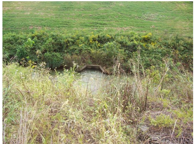
Photo 10 Typical view showing fair conditions of the south fly ash pond discharge structure. Additional mowing is scheduled to be performed within this area.
