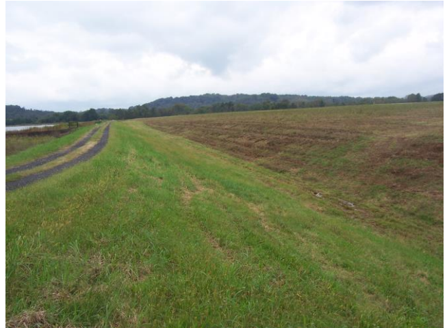
Photo 8 Typical view showing good conditions of the north embankment showing a uniform slope and a well maintained vegetative cover.
