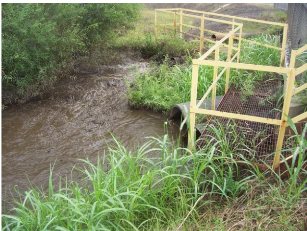
Photo 5 Typical view showing good conditions of unobstructed discharge into the south fly ash pond.
