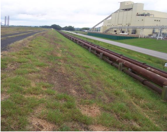
Photo 7 Typical view showing good conditions of the east embankment showing a uniform slope and a well maintained vegetative cover.
